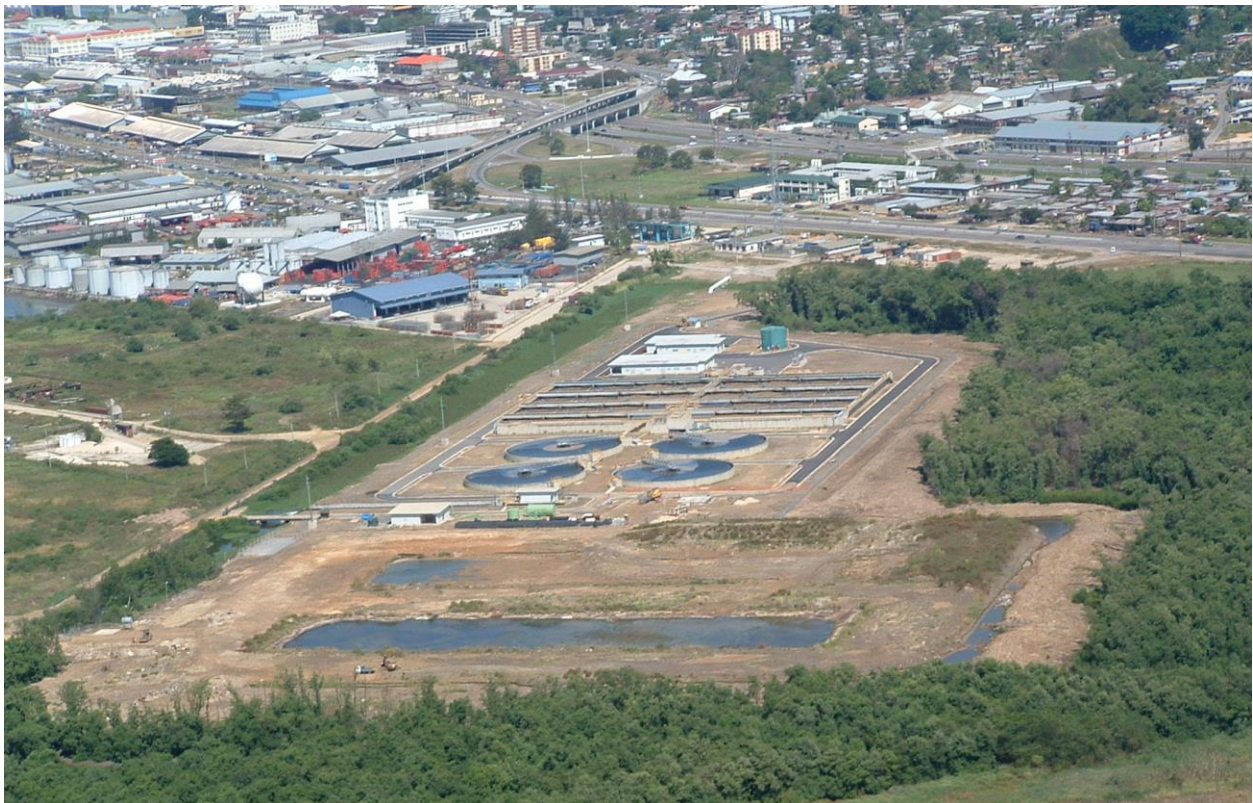
Figure 3: Aerial view of the Beetham Wastewater treatment Plant
